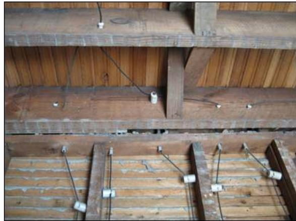
Older wiring systems were not designed to handle large loads. The most dangerous concern is new circuits that have been added onto the original wiring, uncovered and overstuffed junction boxes, and open splices or junction boxes in hidden wall spaces. This is where the electrical fires often start.
