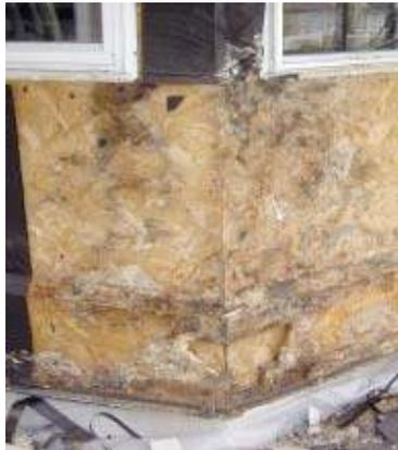
The problems that Mr. McCoy discusses can often be in structures less than two years old. The problems include rotten sheathing and framing members of the exterior walls. All troubles found with manufactured stone are not the result of the stone itself, but due to improper application of the materials.
